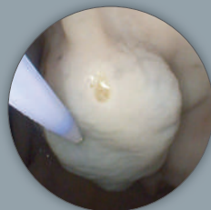
Injection of LiftUp®
